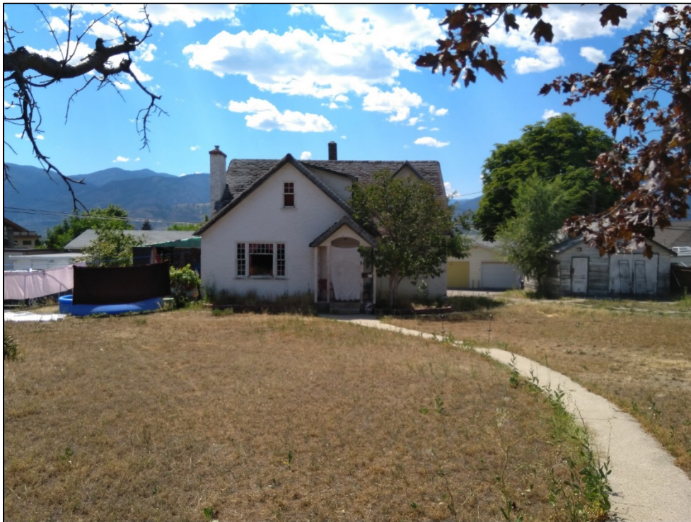
Figure 5: East View of existing dwelling to be demolished
